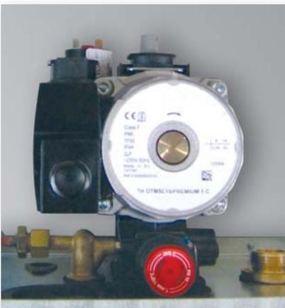
Pump body with built-in air vent
